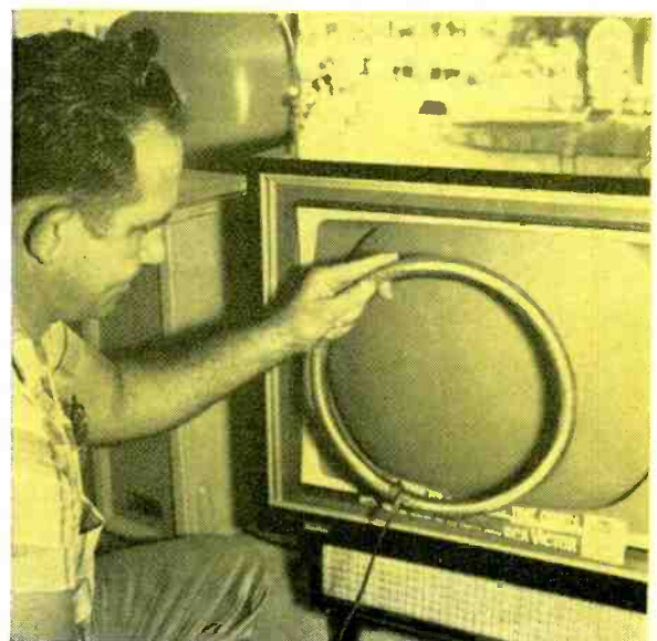
Adjusting height control inside contrast-control shaft.
